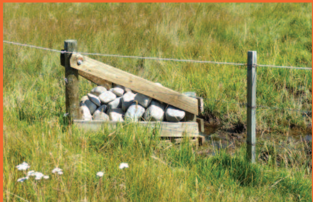
Anchor posts in flood-prone areas with rock or concrete.
